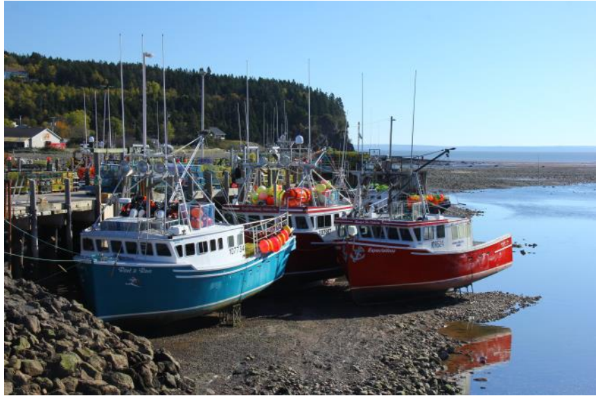
Alma’s harbour will be upgraded over the next two years.
